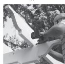
**17.** Continue working out from the center until the rafters are installed.
