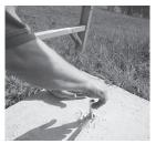
**5.** Use the 15/16" socket wrench to tighten the nut on top of the anchor.
