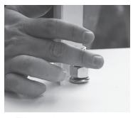
13. Tilting the column to one side may make it easier to position the rod so it can be inserted through the hole in the cap. Make sure that the attached angle is oriented properly. Caulk around the center hole. Only finger tighten the stainless steel nut at this time.
