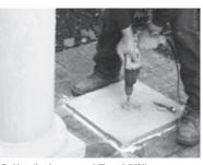
2. Use the hammer drill and 5/8" masonry bit to drill a 5" deep hole.
