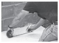
1. Locate the center points of the columns. Make sure the layout and slab are square. NOTE: The concrete slab needs to be a minimum of 5" thick. The concrete footing must be a minimum of 2'x2'x2' and needs to reflect the local building code requirements. Concrete must be a minimum of 2,000 psi.
