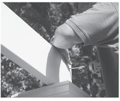
**14.** Install all the headers without decorative rafter tails to the outside of the aluminum angles on top of the columns using the 2.5" hex head stainless steel screws. Set the clutch on the drill so the screw is not stripped.
